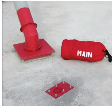
Concrete anchor plate developed by Edon Farmers Cooperative and Scott Equity Exchange, in conjunction with SATRA. Anchor plate is color-coded red for main line or blue for belay line.
