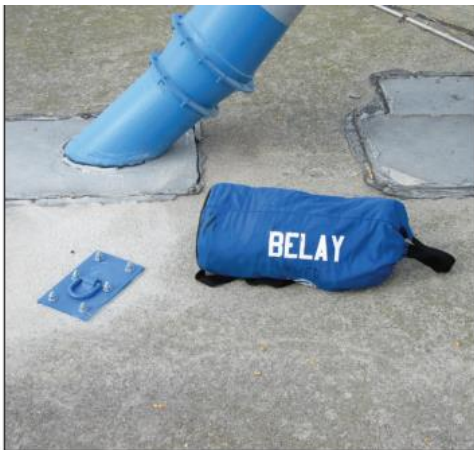
Concrete anchor plate developed by Edon Farmers Cooperative and Scott Equity Exchange, in conjunction with SATRA. Anchor plate is color-coded red for main line or blue for belay line.
